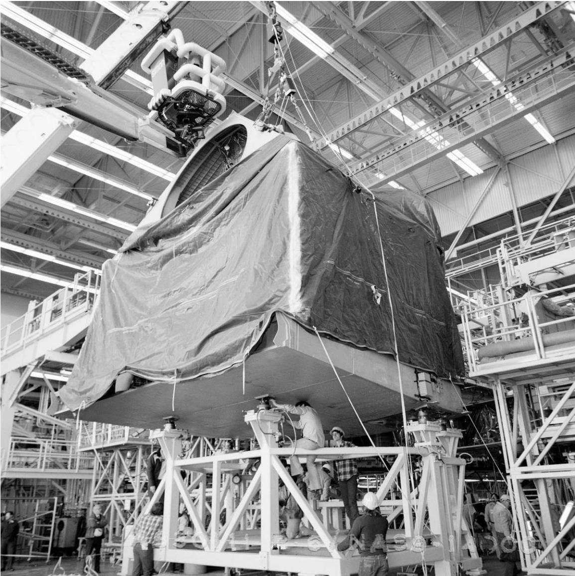
Figure B-36. Preparing for the installation of Discovery's aft fuselage in High Bay 2, AFP 42, January 11, 1983.
